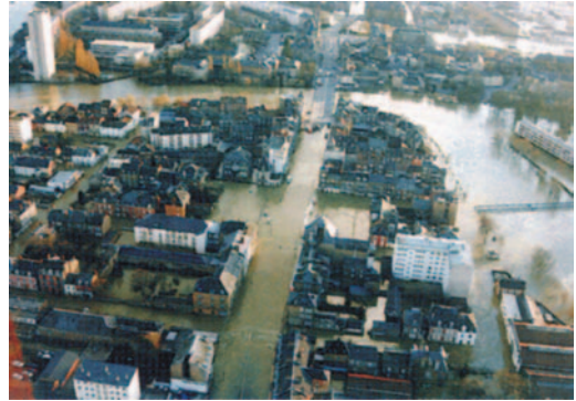
Figure 3. The 1995 flood in Charleville-Mézières (Ardennes, France).
